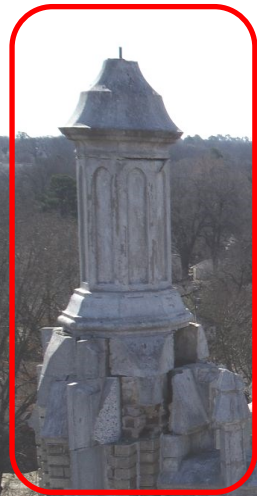
February 2022 Lightning Strike Damage to Belltower
